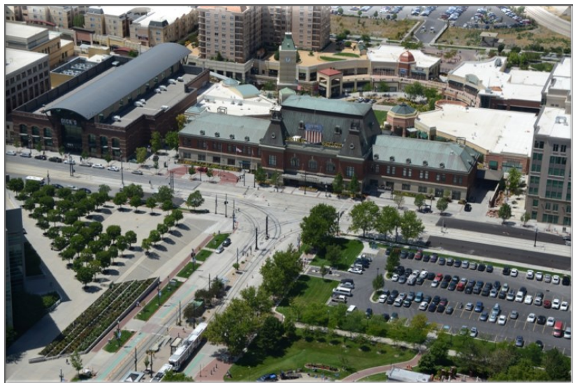
Half Grand TRAX Airport Line tie-in track complete in anticipation of opening of airport line in April 2013
