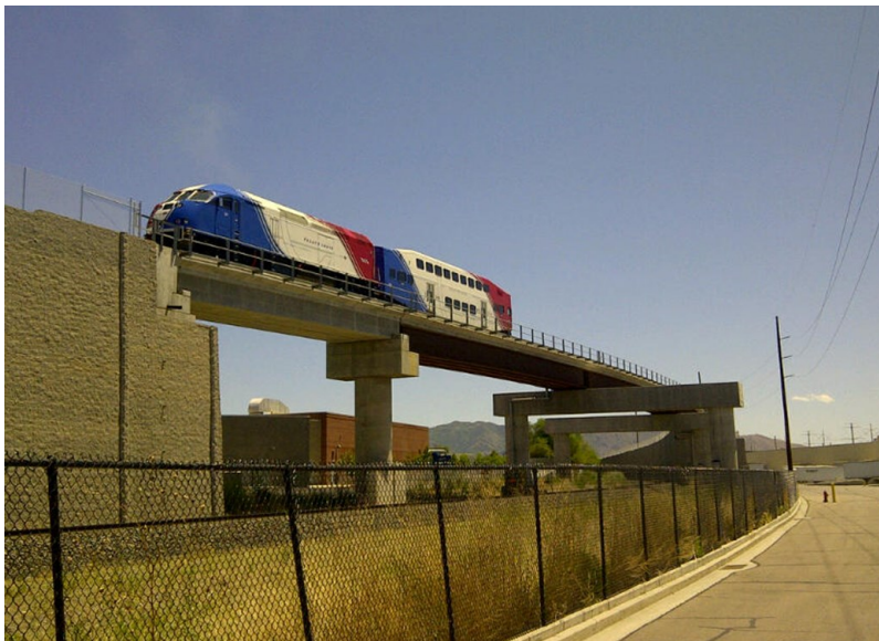
South Jordan Overpass and FrontRunner South
